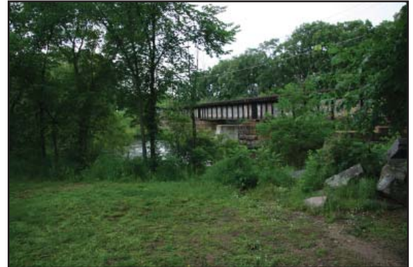
The existing Sauk River railroad bridge.
