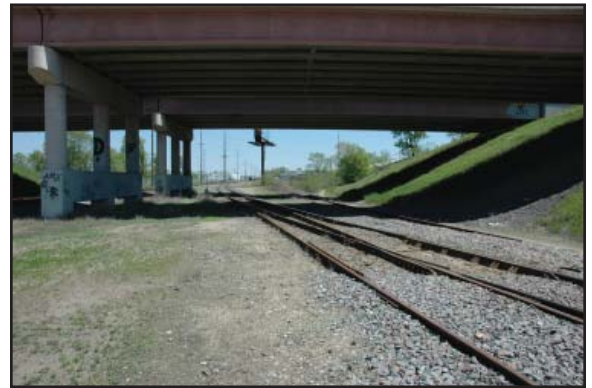
The railroad corridor under the State Highway 15 Bridge.
