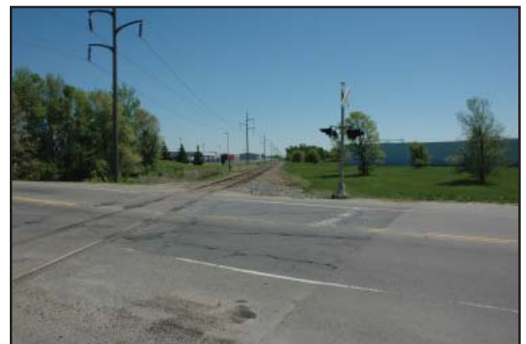
Road crossing at Saukview Drive.
