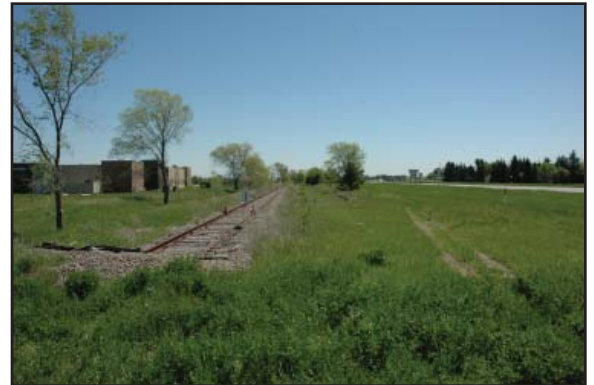
The proposed trail will utilize the existing rail bed just east of CR 133 in St. Joseph.
