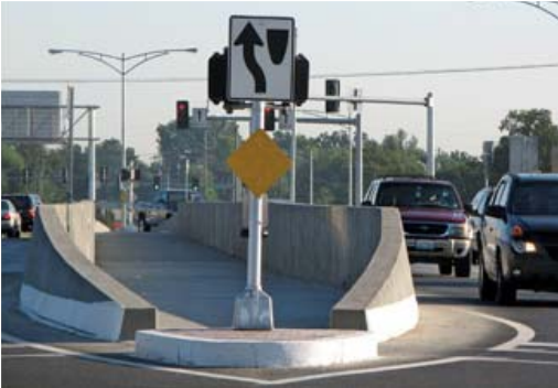
Pedestrians cross the bridge using a center island.
