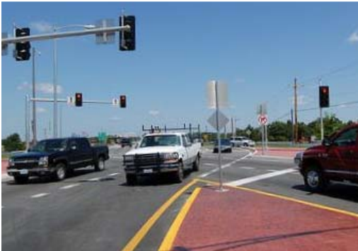
Traffic crisscrosses at either end of the bridge, so instead of making hard left turns, drivers veer to the left for access.
