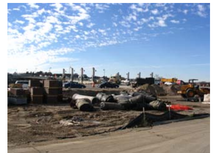
Sauk Rapids Bridge and Benton Drive under Construction Fall 2007
