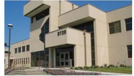
TAC Meeting Location: Mn/DOT District 3 Building
